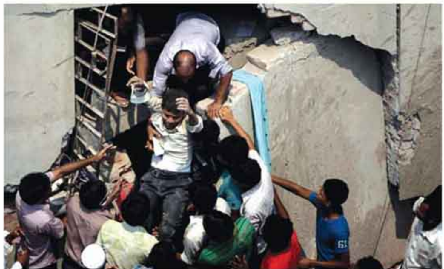
An injured is rescued from the collapse
